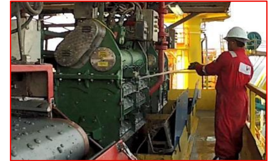
Washing plugged screens
